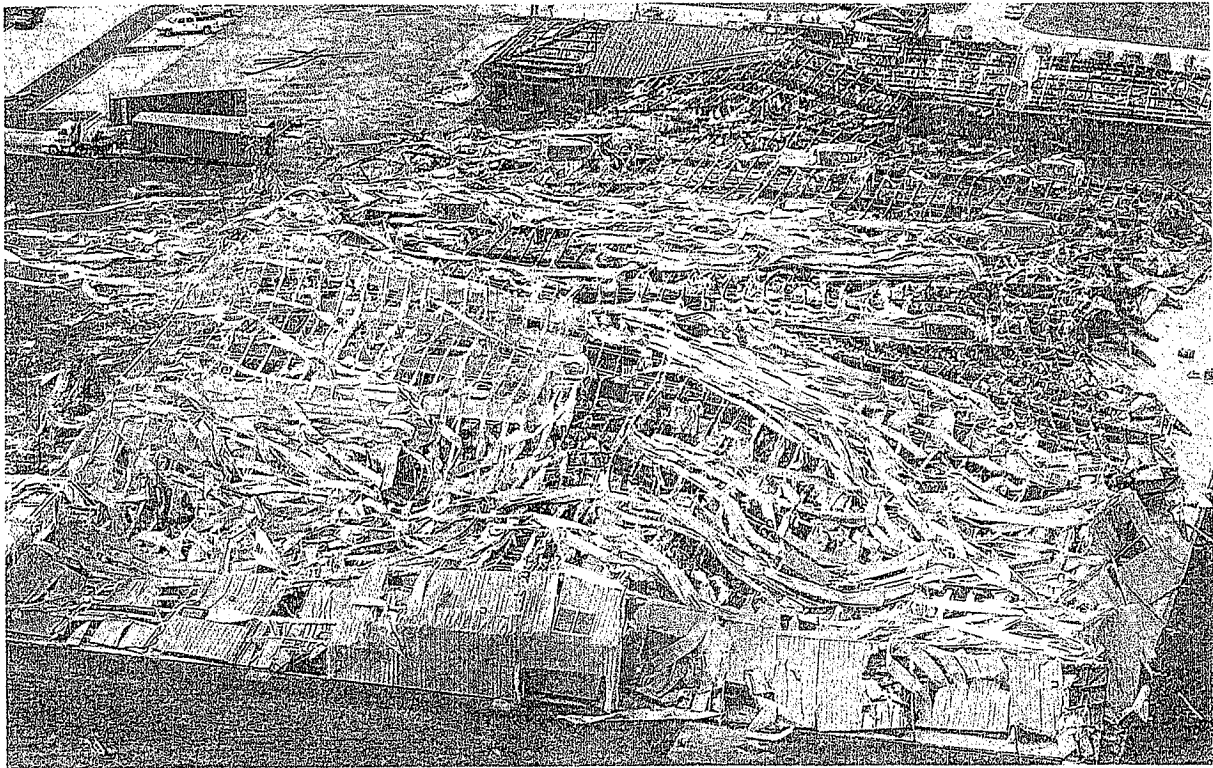
OKLAHOMA CITY, 2003 This factory was leveled by a tornado on May 9; the storm's path of destruction stretched for 35 miles
